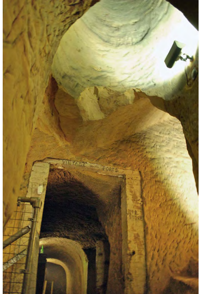
Junction with stairs down (left), entrance to vintage ports gallery (middle), stairs up to the likely original entrance (right) – and above them all the shaft of the largest of the three wells, which appears at every level of the caves
